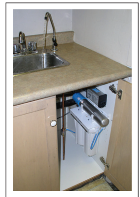
Typical Installation for drinking water under the sink
